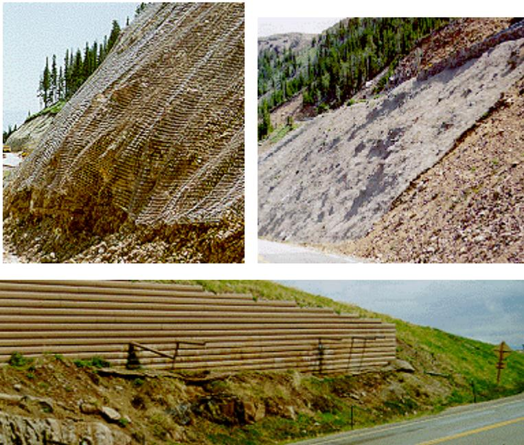
Figure 6. Slope-stabilization methods. Chicken wire (top left) and concrete (top right) cover exposed slopes and a retaining wall with drainage pipes protects the road (below). All images from the Rocky Mountains.
